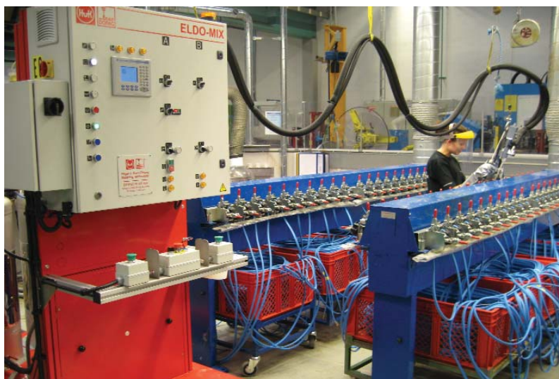
The SQFlex pump plug encapsulating facility
