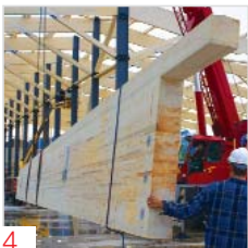
4 Fixing the roof
