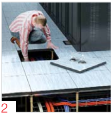
2 Under floor access
